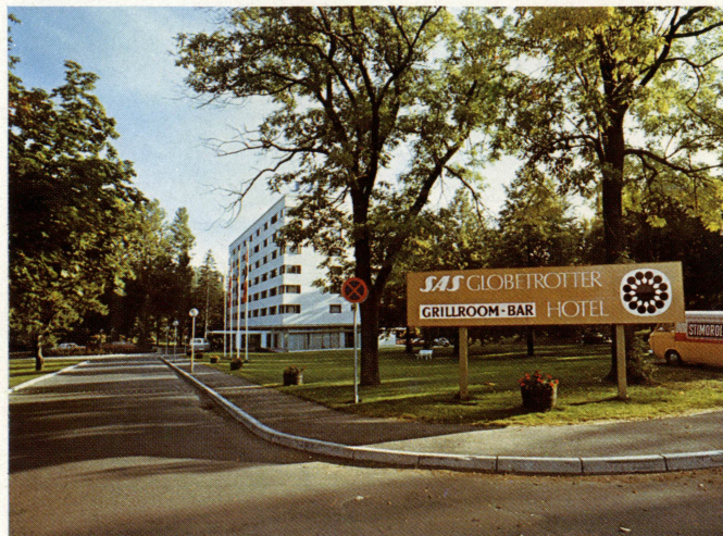
The SAS Globetrotter Hotel near Oslo's Fornebu Airport provides both first class rooms, restaurants and congress facilities.
